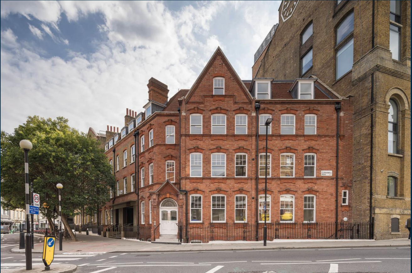
The Skipper Building, London
